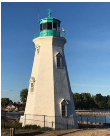
Inner Range Lighthouse 1898 with chainlink fencing
